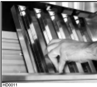
BAFFLE FILTER (TYPICAL)
